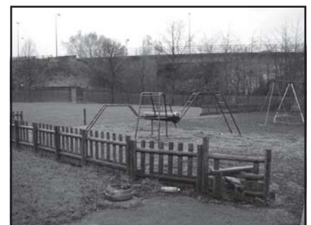
Spider Park before the repairs
